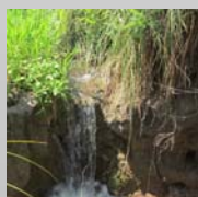
Headcut at site F2
