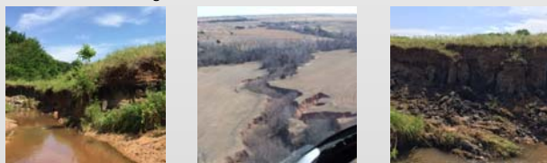
Unstable channels in the Fort Cobb Reservoir Watershed contribute a significant amount of sediment to the reservoir.
